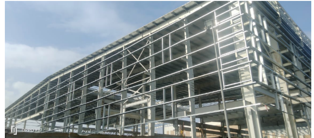
Khatalwada plant expansion building
