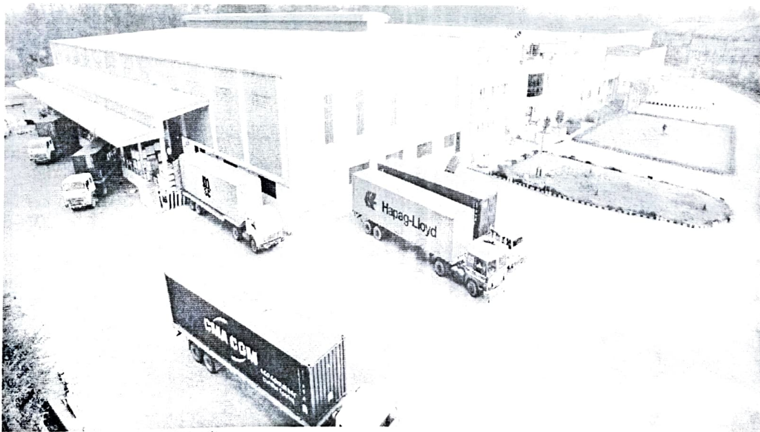
Above: photo of the Silvassa Facility.
